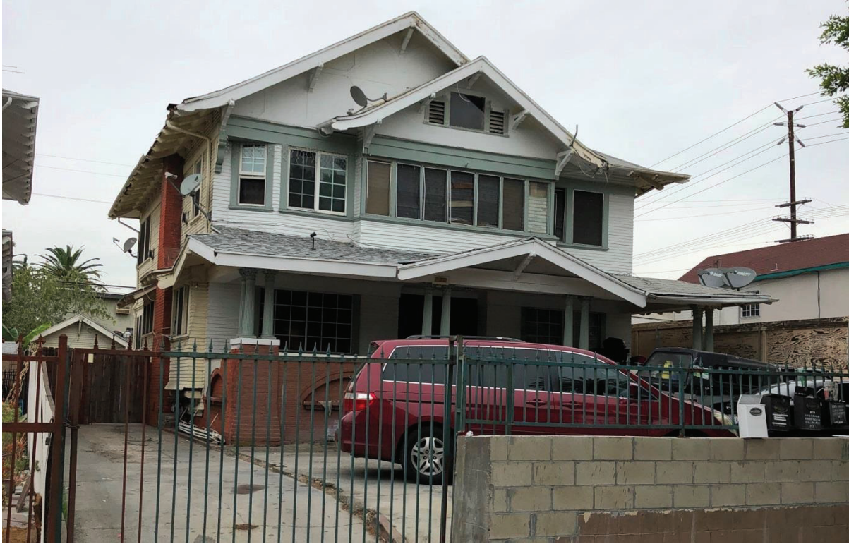
Figure 11 1033 North New Hampshire Avenue, East and South Elevations, View Northwest
