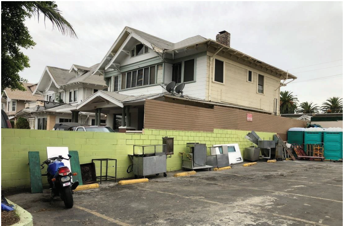
Figure 12 630 North Oxford Avenue, East and North Elevations, View Southwest
