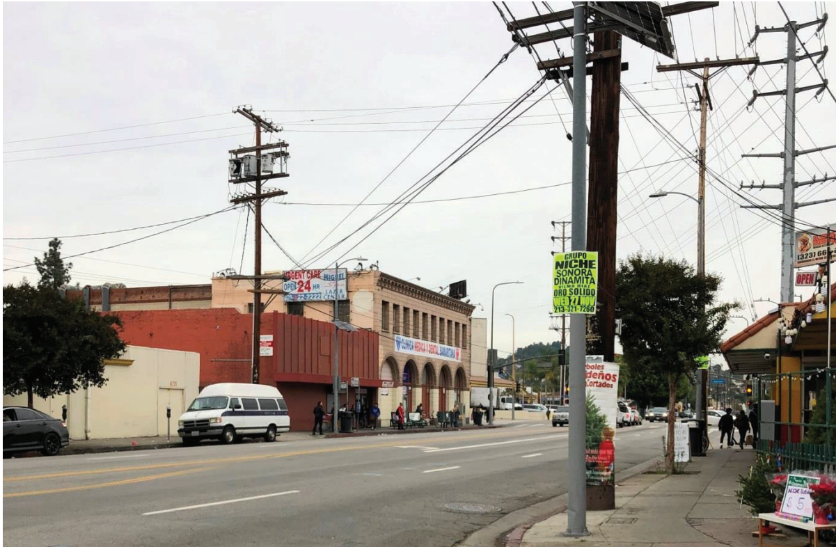
Figure 8 4700 Block of West Santa Monica Boulevard, Facing Northeast
